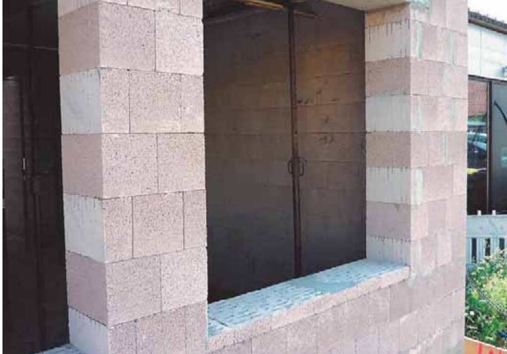
Photo 8: maçonnerie en parpaings plans (Photo: Bisotherm GmbH, Mülheim-Kärlich).
